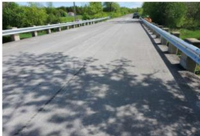
Photo 3: Asphalt on Concrete Deck
