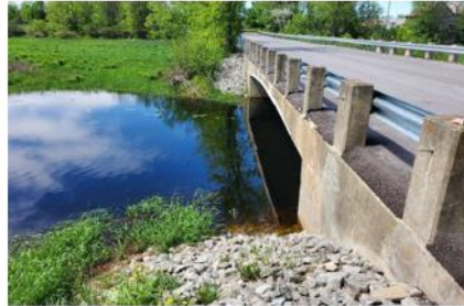
Photo 2: West Elevation Looking South
