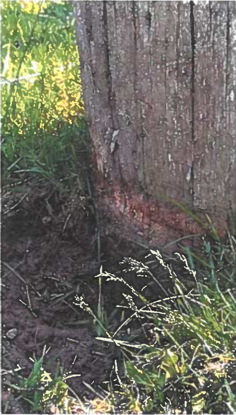
Divots taken to assess below grade condition. Treatment is visible
