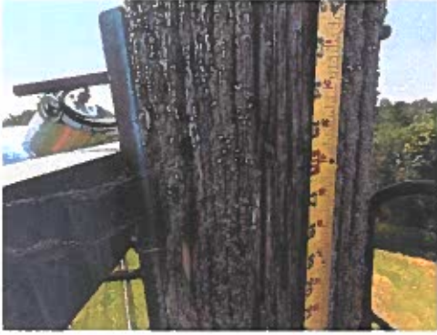
Light fixture mounted at 16" from top of pole
