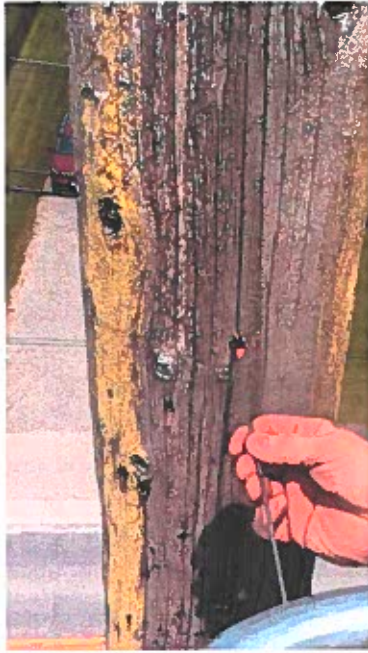
Shell thickness reading conducted at roof section of right field pole
