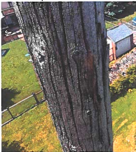
External void exhibiting approximately \frac{3}{4} " Depth 2.5" wide
