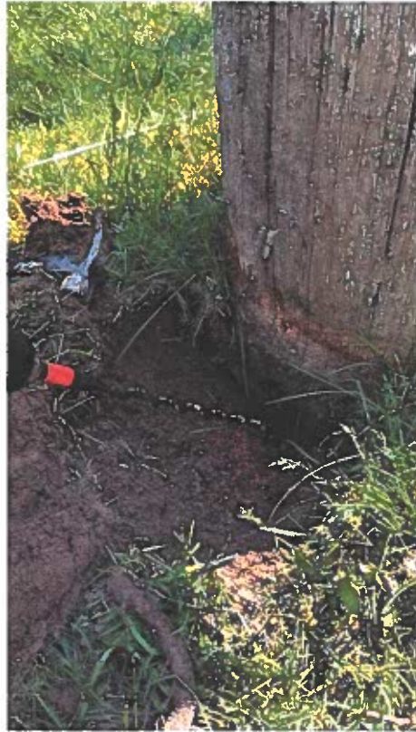
Boring below grade to conduct shell thickness reading
