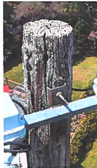
Upper roof portion of left field pole indicating light to medium weathering
