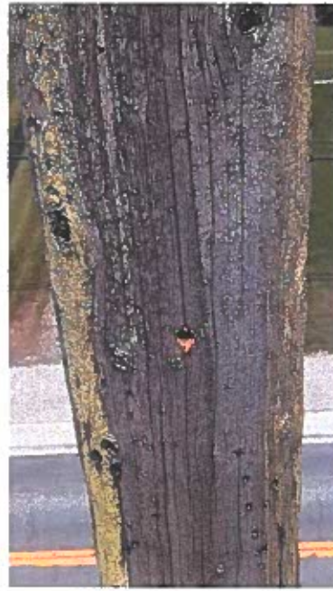
Bore hole at roof section of right field pole
